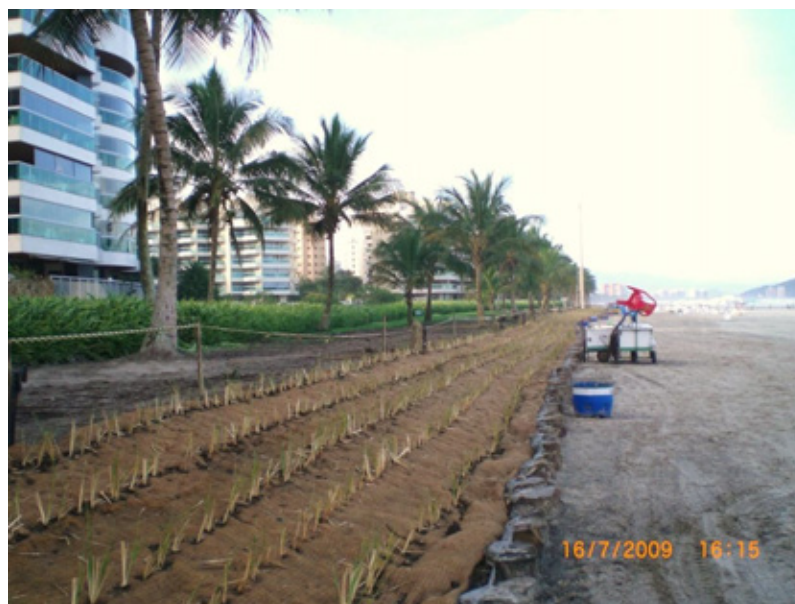
Figure 12: Final Project executed: palisade, erosion control blanket and Vetiver hedgerows. Source: Luiz Lucena.
