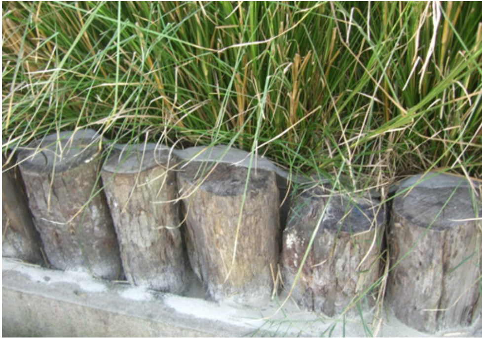
Figure 16: Detail: palisade, geotextile and Vetiver. Source: Luiz Lucena
