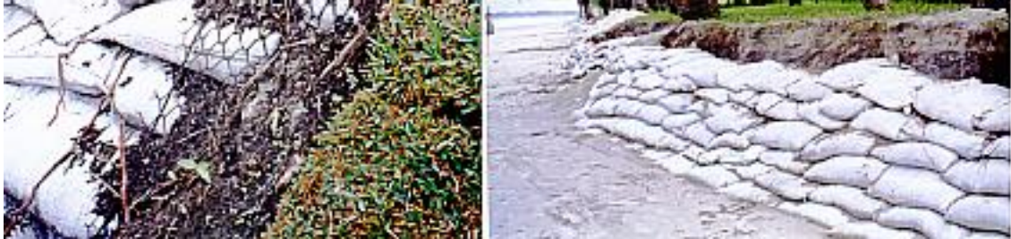
Figure 9: raffia bags to resist surf erosion.
