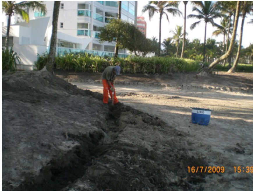
Figure: 19: Trench excavation for sediment retainer installation. Source: Luiz Lucena
