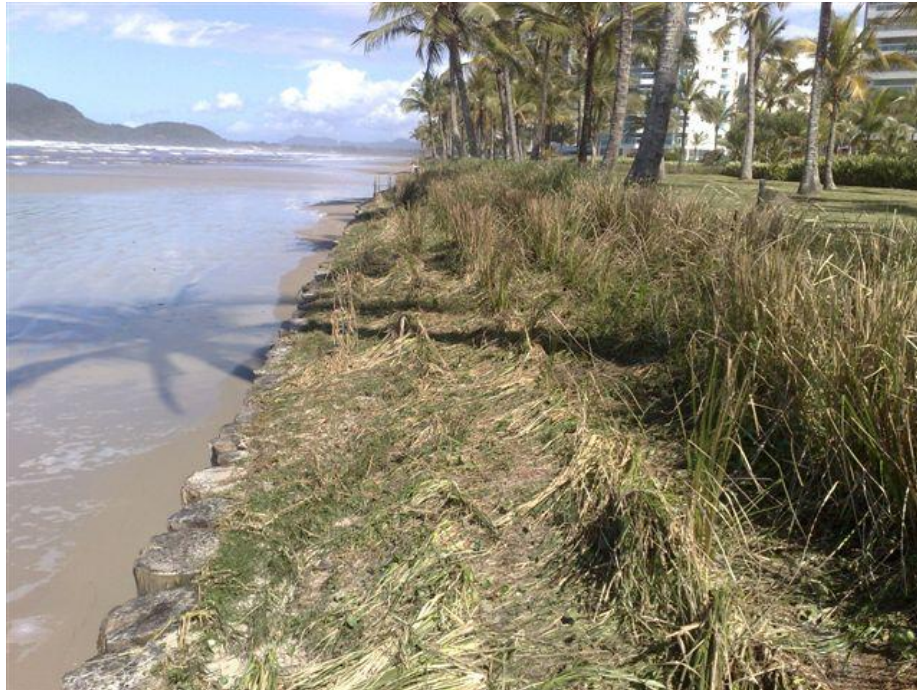
Figure: 24: First 3 Vetiver hedgerows at the worst spot where wave hit and no soil loss observed. Source: Luiz Lucena
