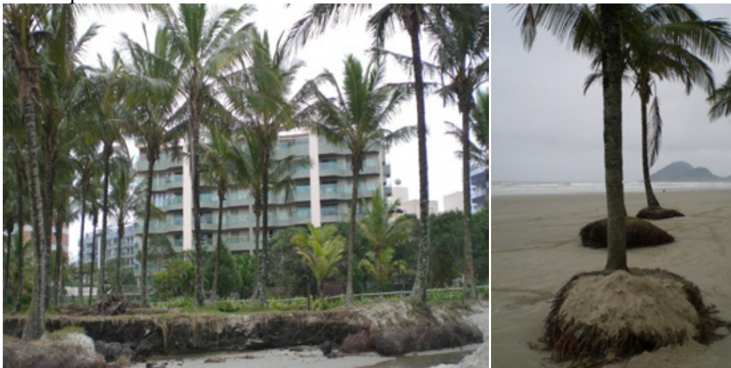
Figure 8: Coastal erosion caused by storm surges and tidal changes.
