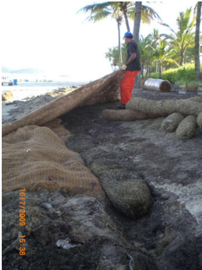
Figure: 20: Installation of erosion control blanket.. Source: Luiz Lucena
